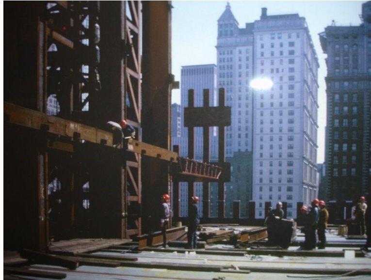
Figure 20: Photo showing a channel with floor truss seats. A floor truss connecting the channel to a perimeter column is shown at the far end of the construction zone.
