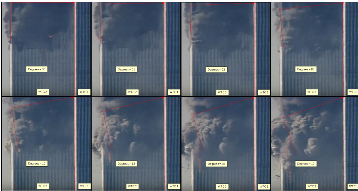
Figure 32: Rotation of the top block of the South Tower suggests a pivot point approximately marked at the circle.
