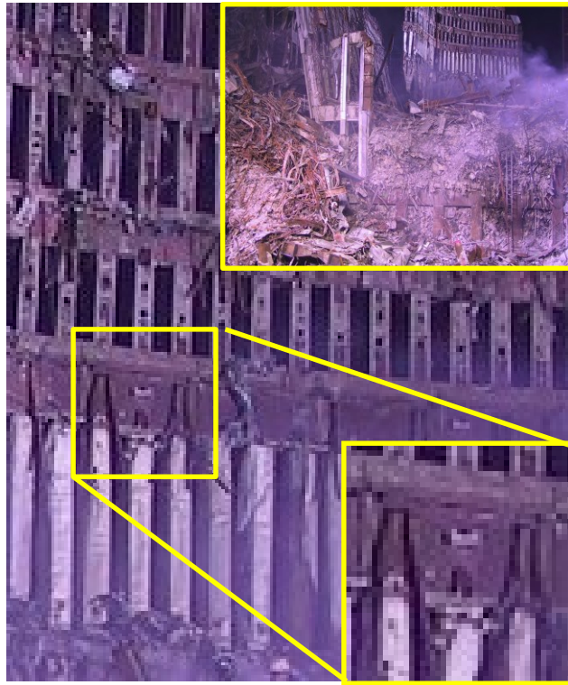
Figure 46: Inner perimeter columns in "Zone 3" of the North Tower showing hanging floor truss top chords.
